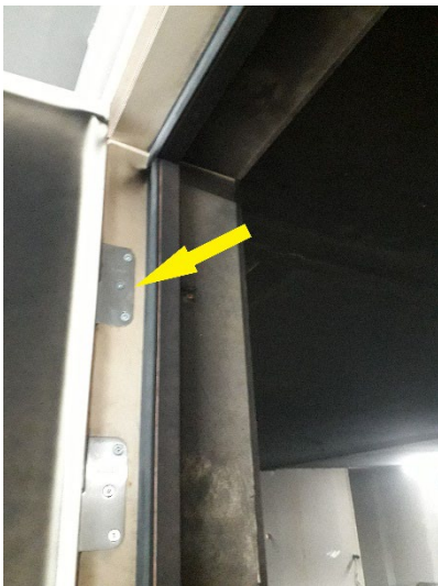
Smoke control door ("clean" frame to the left of the rebate)
