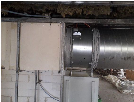
Detail rectangular duct – fan – circular duct
