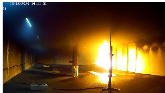
After 3'31" (activation 2 nd sprinkler)
