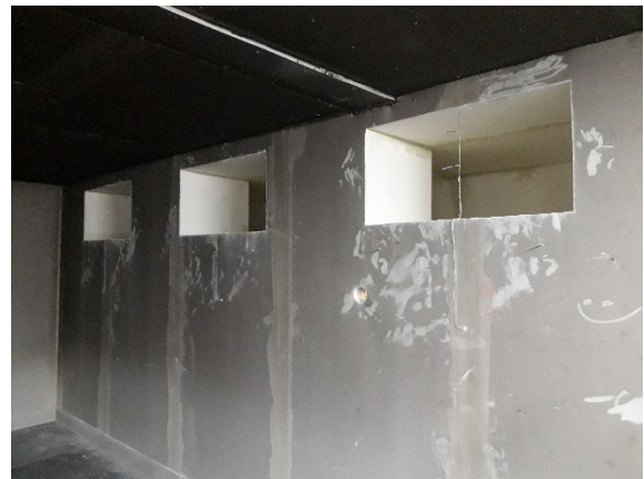
Exhaust openings in the common area
