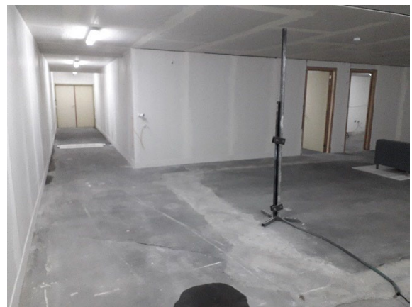
Evacuation route with double door to the end
